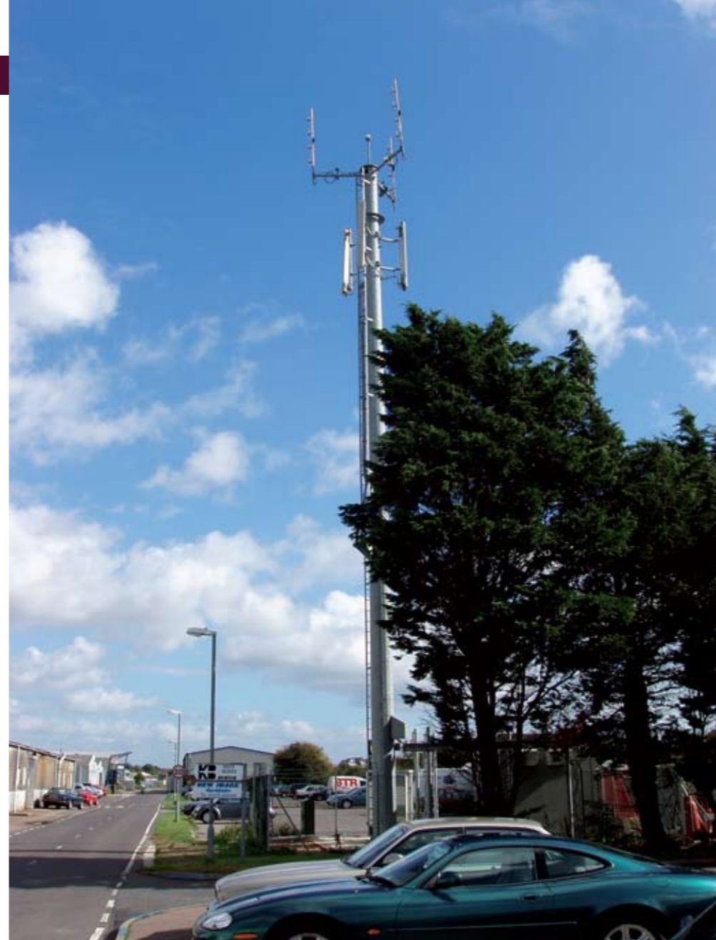
Tetramast i West Sussex, England.
